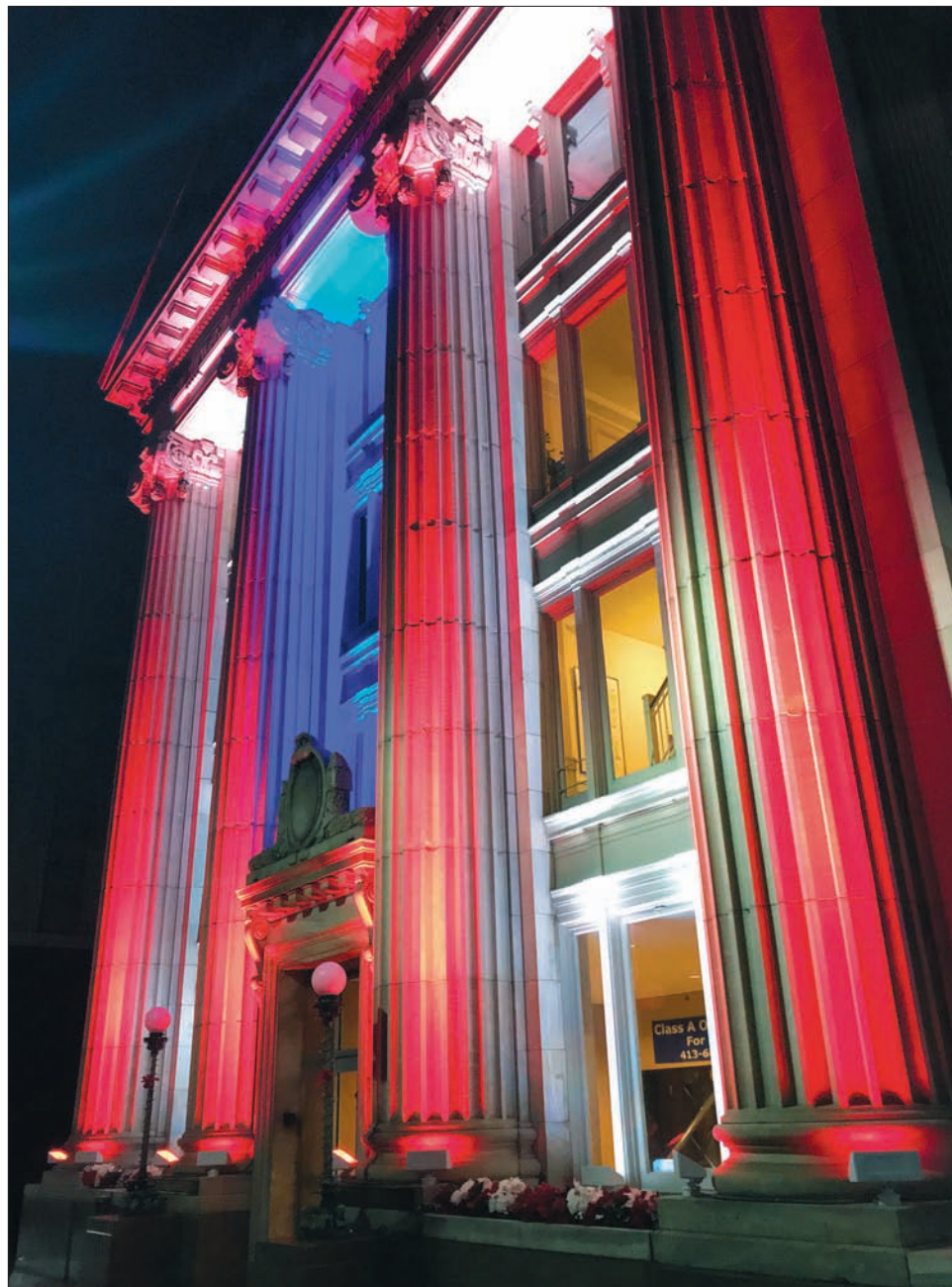
On each night since the winter solstice, the facade of the building at 100 North St. in downtown Pittsfield has been bathed in colorful changing lights positioned to highlight its architectural features. The high-tech lighting display is part of a demonstration project by Berkshire Lightscares, which hopes to encourage permanent lighting displays at other downtown buildings and public spaces. (Photo by Cody Johnson)
